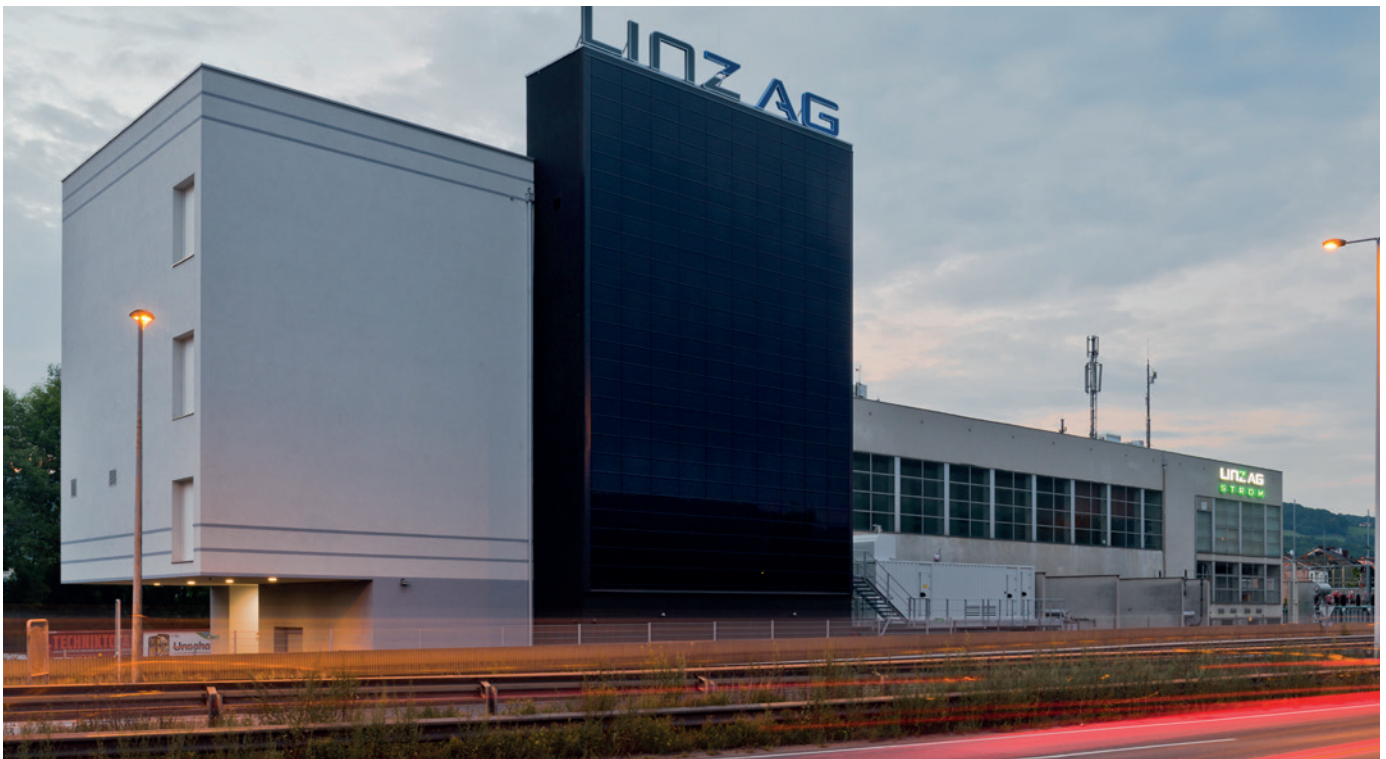
Data Center 2 Linz AG, AT (Planung: BHM-Ingineure, Linz, AT; Produkte: StoVentec Photovoltaics Inlay, StoTherm System; Foto: Christian Schellander, artboxx)
